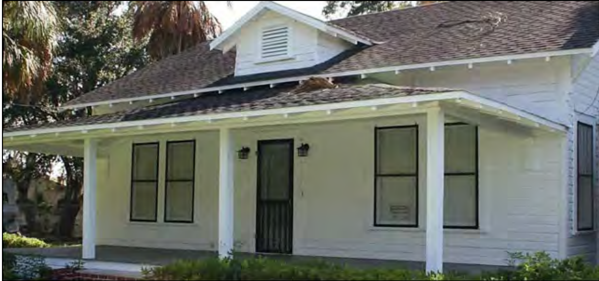
Photo 5-15: Aaron E. and Maude Morgan House, west front and south side elevations showing German siding and Craftsman-style windows, door, and exposed rafter tails, 2020.
