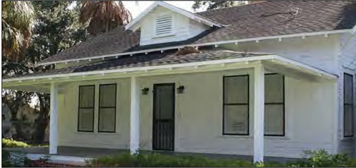
Figure 2. Aaron E. and Maude Morgan House: west front and south side elevations showing German siding and Craftsman-style windows, door, and exposed rafter tails, 2020.
